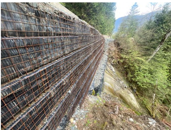
Wall facing and gabion foundation
