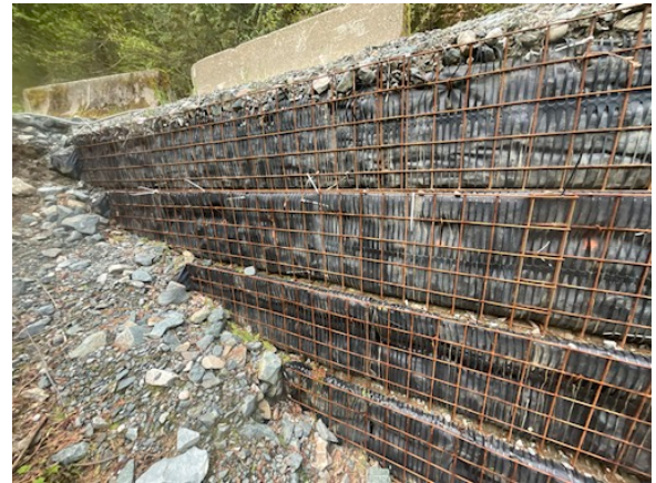
Geosynthetic and welded wire mesh
